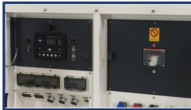
REAR CONTROL PANEL WITH MLCB
